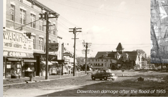
Downtown damage after the flood of 1955
